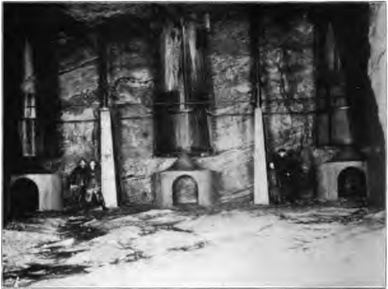
VICTORIA HYDRAULIC COMPRESSOR. Lower End, Showing Deflectors. (Water Line Is One Foot Above Cylinder Extension of Shafts).
